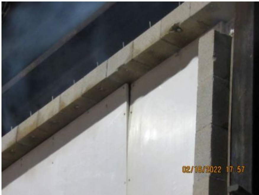
Photo No. 12 Wall popping out at joint continued
