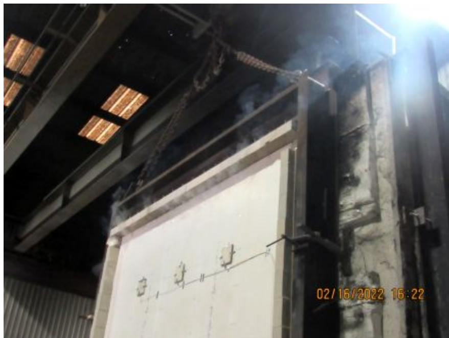
Photo No. 8 Steam from top of wall
